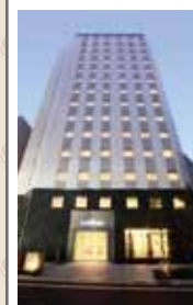
The landmark white 14-story building
